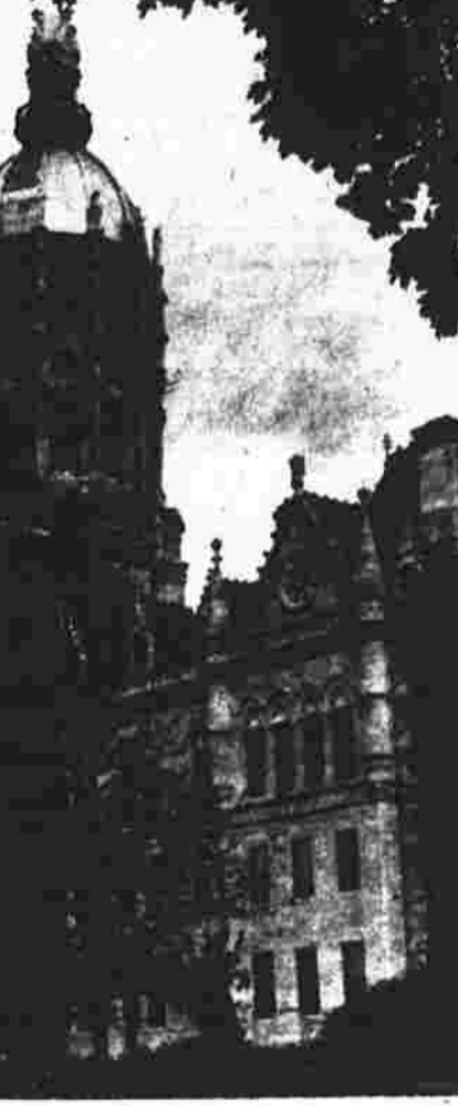
Clean and shiny — The south-east section of the Connecticut State Capitol in Hartford, is exposed for the first time in nearly two years as almost $1 million worth of scaffolding starts to come down as the $8.85 million exterior restoration project of the 101-year-old building draws to a close. (UPI photo)
